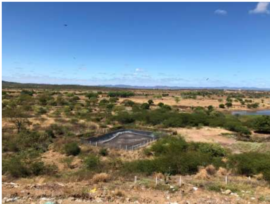
FIGURE 06: Slurry collection tank.
