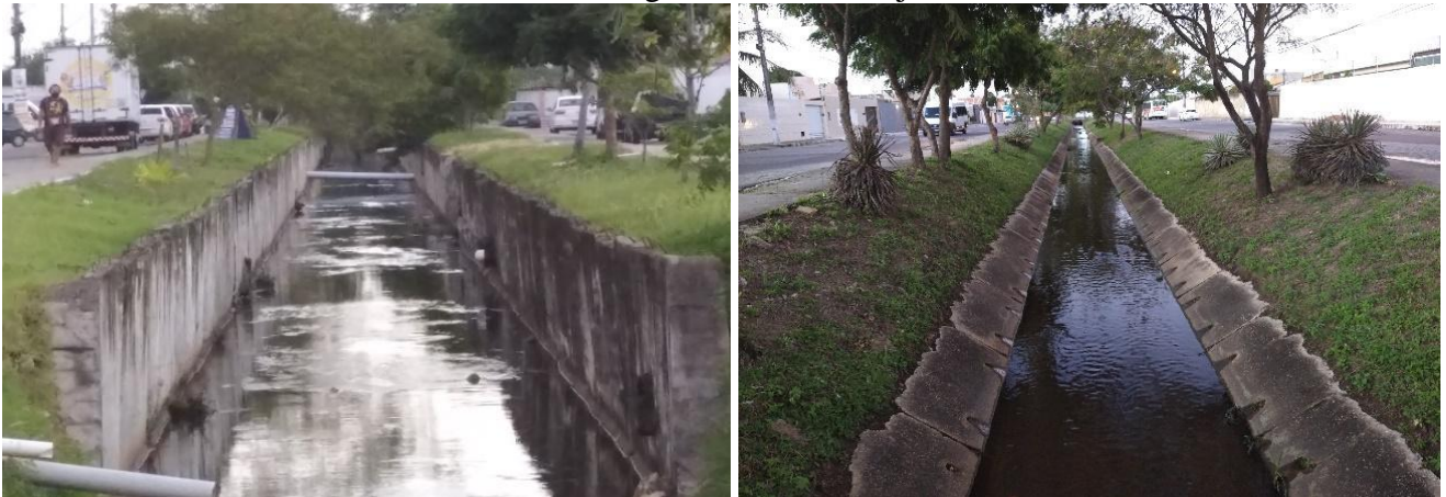
FIGURE 02: Rectangular section (left) and trapezoidal section (right) of the urban drainage channel in the Aruana neighborhood, Aracaju-SE.
