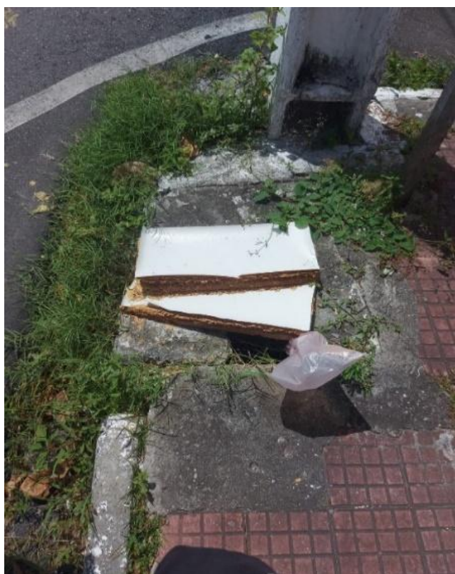
FIGURE 06: Example of poorly located and badly maintained gutter inlets.
