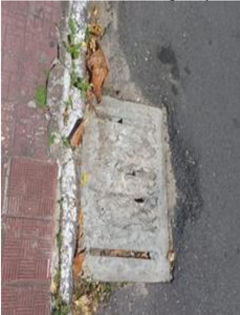
FIGURE 08: Gutter inlet completely blocked.
